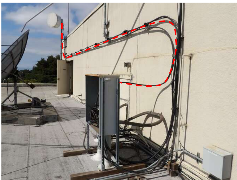
Antenna Waveguide Photo
