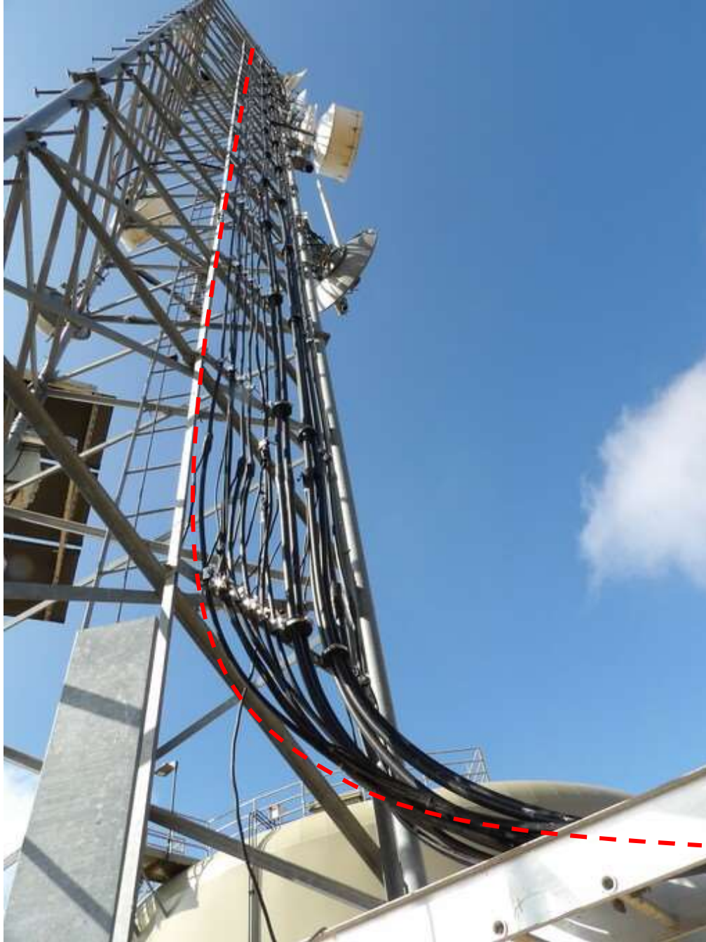
Antenna Waveguide Photo
