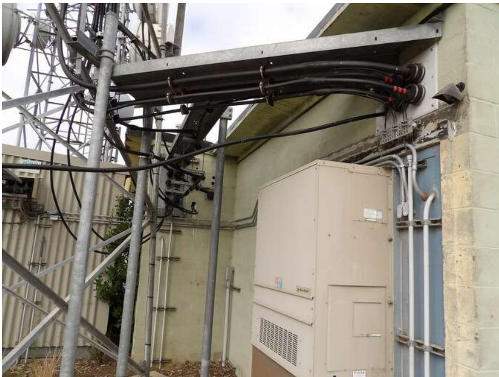
Antenna Cable Ice Bridge
