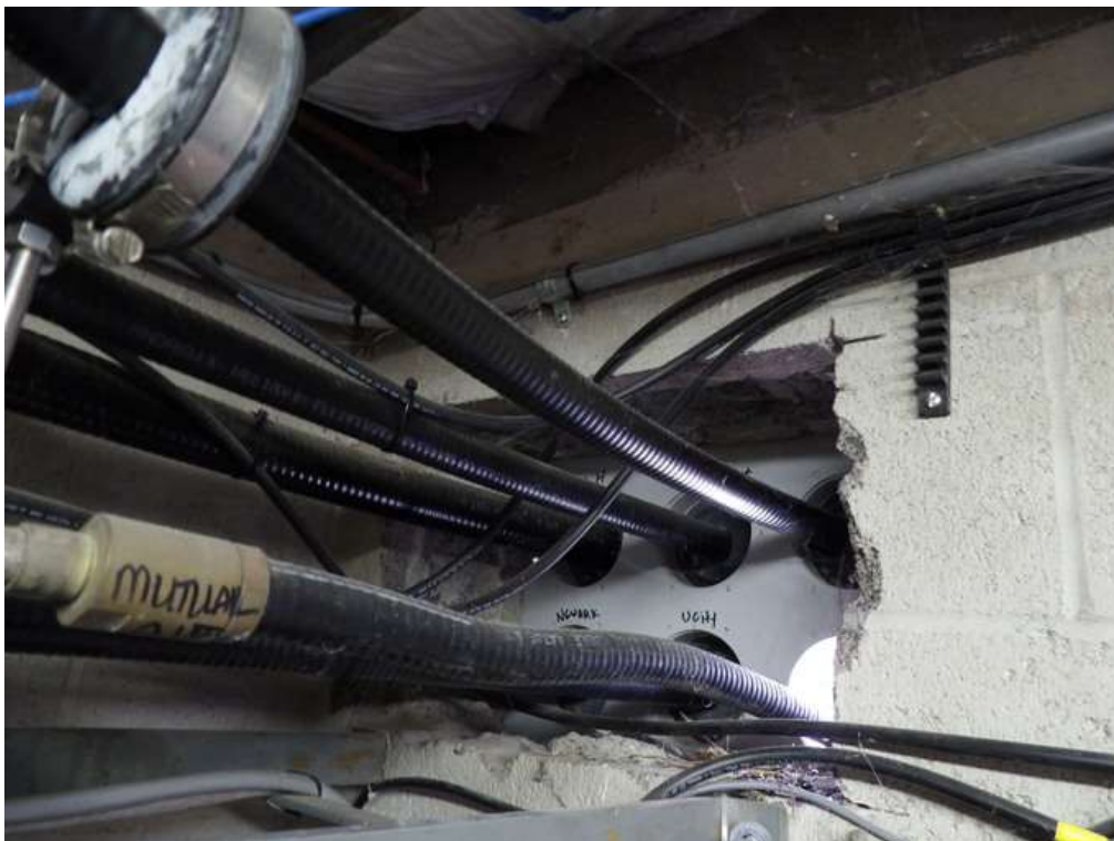
Antenna Interior Entry Port
