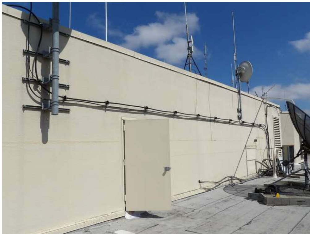
Antenna Cable Ice Bridge
